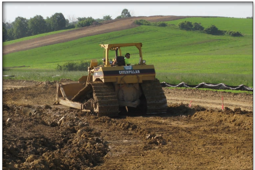
BUTLER RIDGE WINDFARM Iron Ridge, WI
